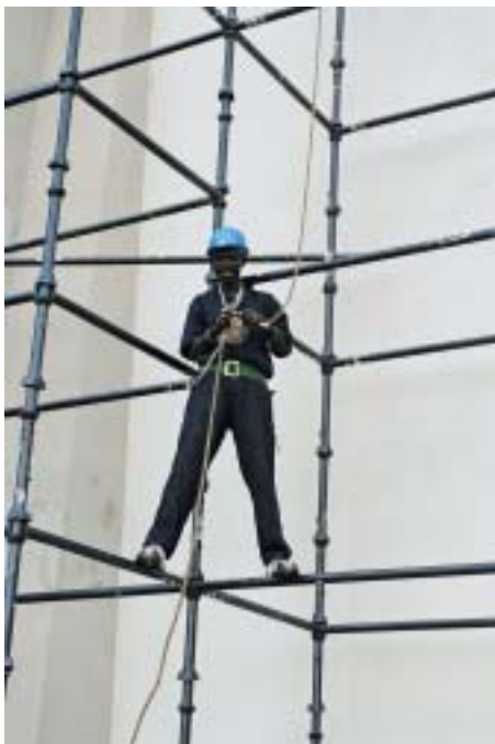
Construction: Reconstructing the facade of St. Joseph's Cathedral - Dar Es Salaam, Tanzania.
